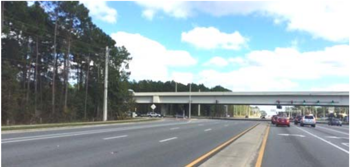
The subject site on the left facing east on Beach Blvd
